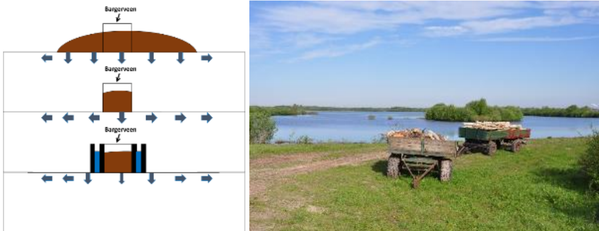
Fig. 5: Left: Restoration of parts of the Bargerveen (Netherlands) by compensating for the loss of large parts of the original bog dome by constructing huge dikes and water storage basins. 61 Right: One of the storage basins with surrounding dikes.
