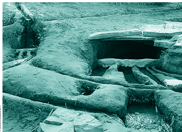
The complex, cooperative water management system for maintaining the fouggaras , human-made underground water systems, has assured water supplies to oases in Algeria since the 7th century.
