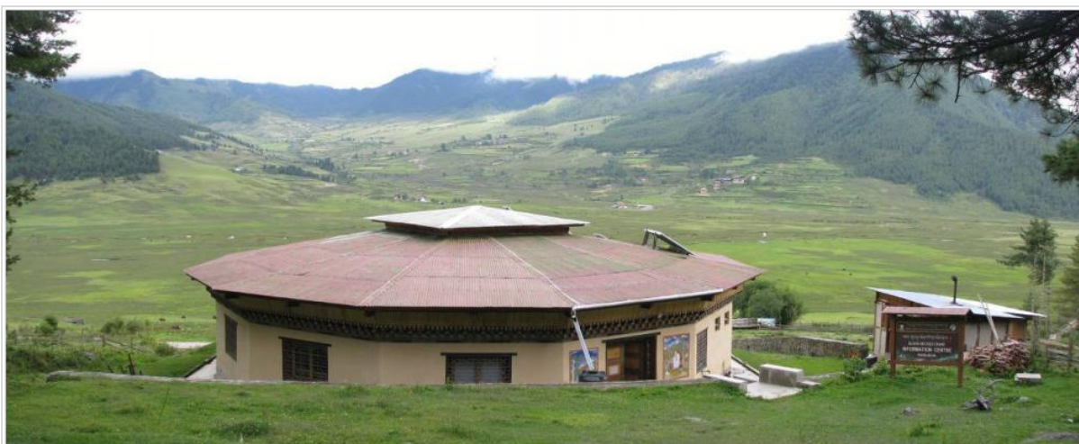
Black-necked Crane Information Centre – Royal Society for the Protection of Nature, Phobjikha (Bhutan)
