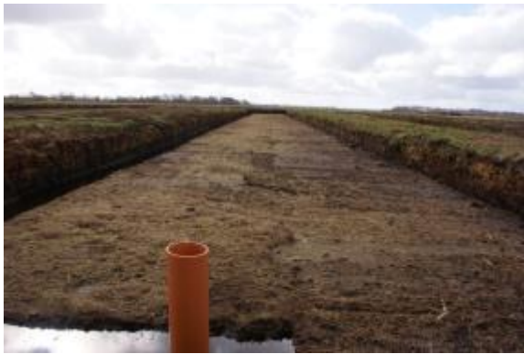
Figure 5.4. Left: A ditch canalizing the water from the inlet down along the restoration plot. Figure on the right is a sketch of how a tube can connect the restoration plot with a nearby ditch to control the inlet of water. The same arrangement can be made in the other end of the plot to control the outlet of water. Photo © Peter Hahn, Lille Vildmose. Denmark. 2013.
