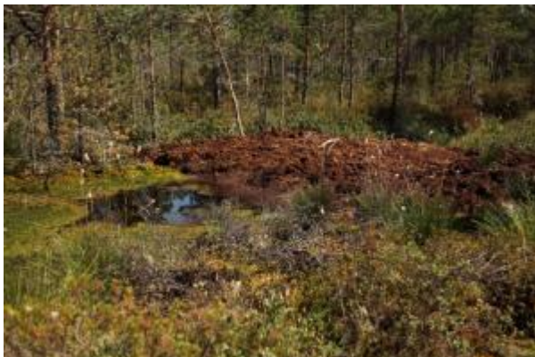
Figure 3.5. Freshly built peat dam. Building of a peat dam is carried out by the excavator, taking the wet peat from the area near the ditch. Dam is built high enough not to have water overflow and wider than the width of the ditch. The operation is closed with covering the compressed peat blocking with the left-over vegetation.
