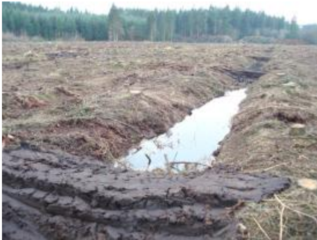
Figure 3.4. Blocking of drainage ditches by peat soil in a degraded peatland. Each blocking is placed for every 10 cm decrease in slope. Pure well-humified peat from the area reachable by the excavator is compressed across the ditch and keyed into both sides of the ditch. In this example peat blocking is used for a 2 meter wide ditch. In areas with a higher slope ditch blocking with peat only is not used if the width of the ditch exceed 1 meter. In such cases other material in combination with peat is needed. Wood could also have been used.
