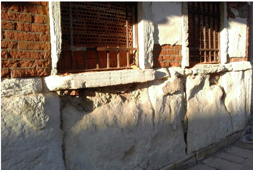
Palazzo Minotto, Fondamenta Briati (Orsoduro 2365-2371A): property of the Commune, closed and with bricked windows, abandoned and out of use since years, with important defects due to humidity (exterior and interior). (Bernhard Furrer, October 2015)
