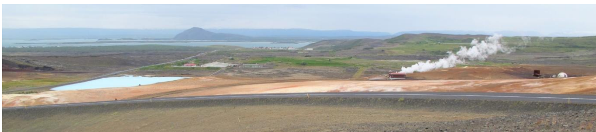
Partial view of the existing Bjarnarflag geothermal plant, its waste water retention pond (left) and Lake Mývatn in the background.
