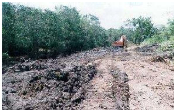
Machinery clearing mangroves at Cuesa River, Chaguaramas by IMA
