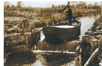
Figure 5b Flap weir (Klappstau) in NW Germany with a fully passable, flexible weir.
