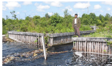
Figure 5a Box block with large spillway, Sebangau NP, Central Kalimantan. Photo © Wim Giesen.
